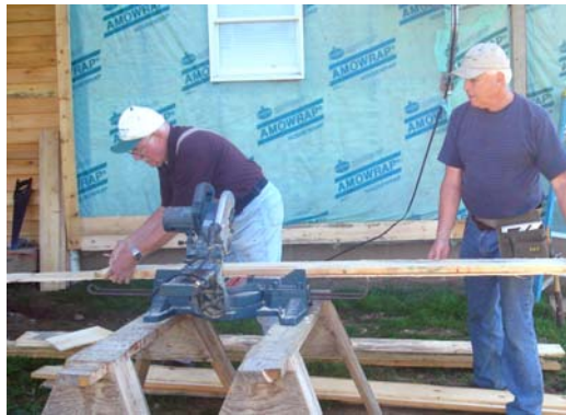
Spence and Barry cutting siding for office building
